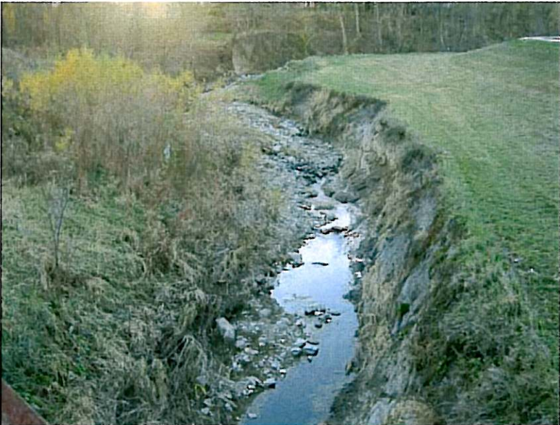
FIGURE 6 Severe Bank Erosion and Incision near Confluence with Big Papillion Creek (looking downstream from golf cart bridge) Whitted Creek Stabilization Study
